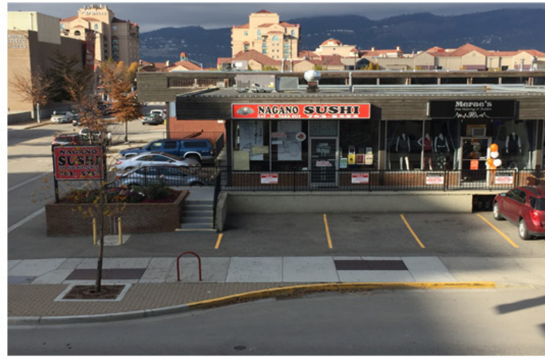
single storey cru
