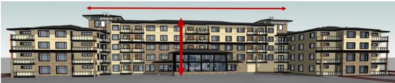
Figure 1 – The red arrows indicate the extent of the requested height variance from 4.5 storeys to 5 storeys for the central portion of the building
