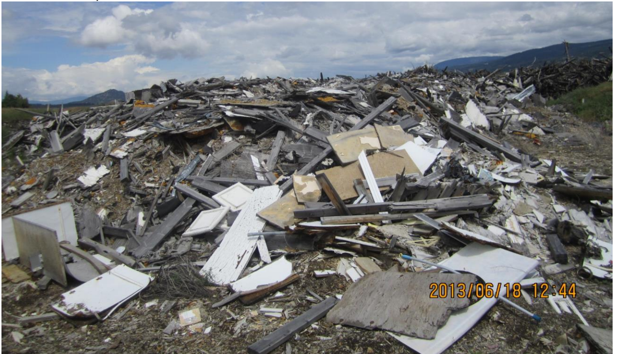
Photo 2. Boards, Metal and Miscellaneous Unsorted Demolition Debris
