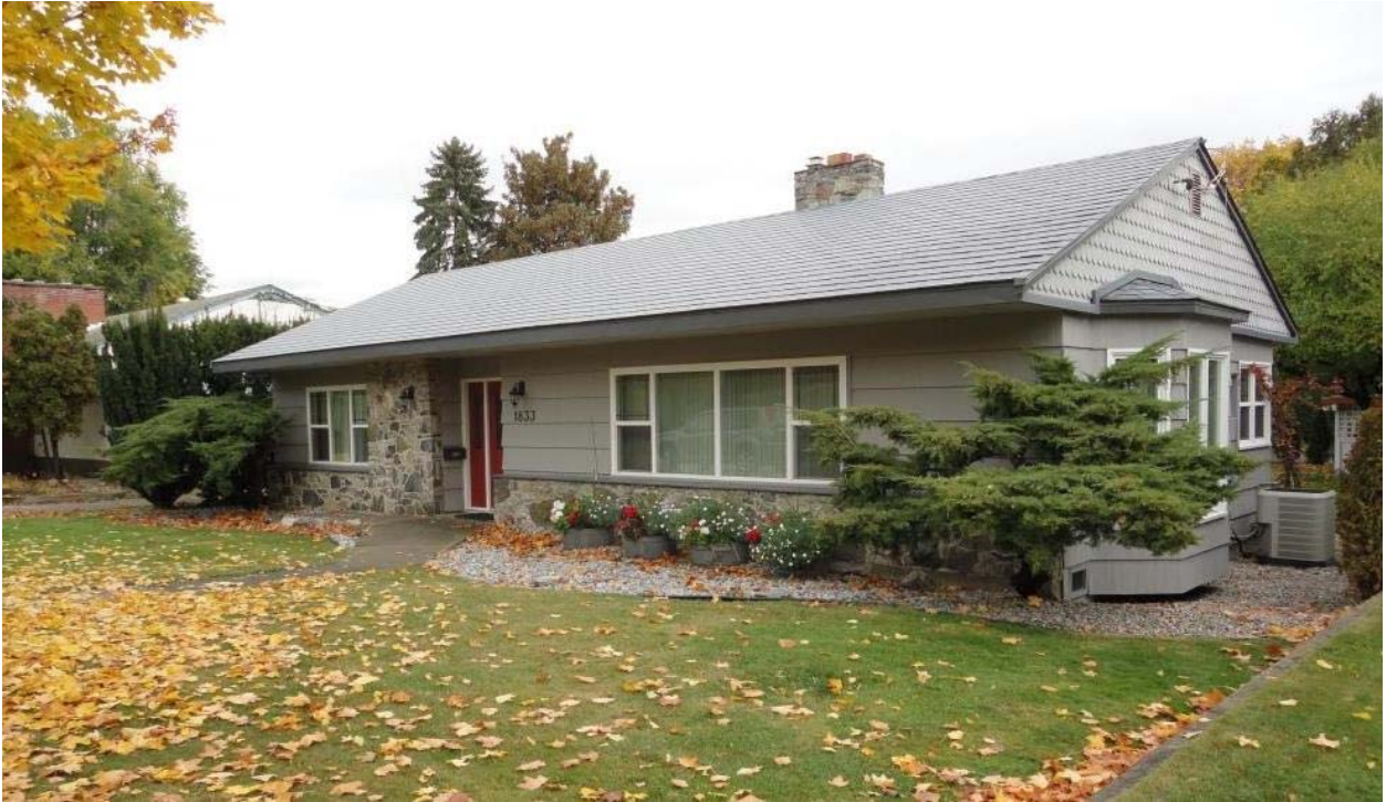
Photo 1: 1833 Abbott Street (before fire). (East side of street).
