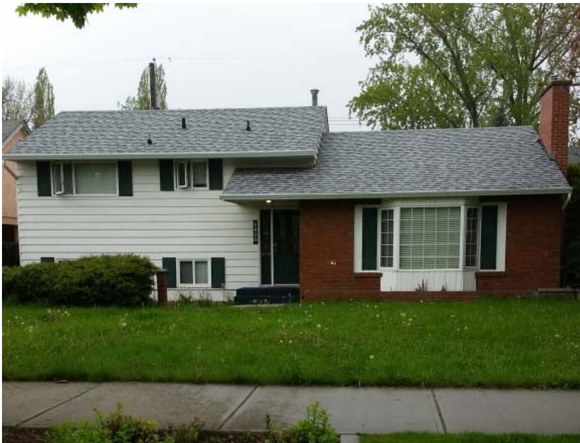
Photo 14: Split level south of house in Photo 13.
