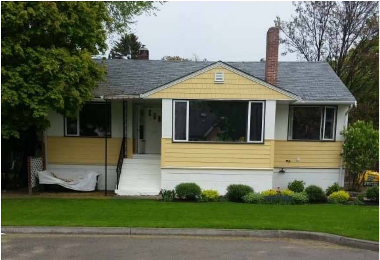
Photo 4: 50's house 2 doors north of house.
