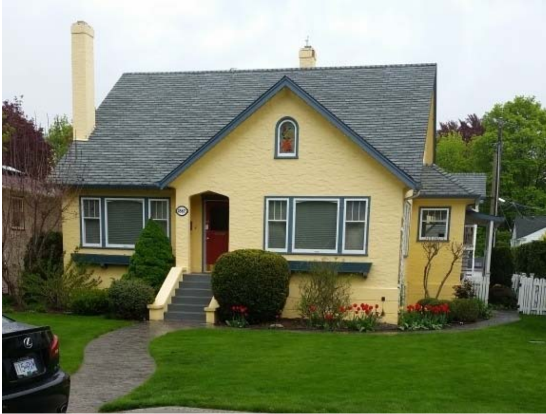
Photo 9: Older character home 4 doors south. (Note front peak and small window in peak).
