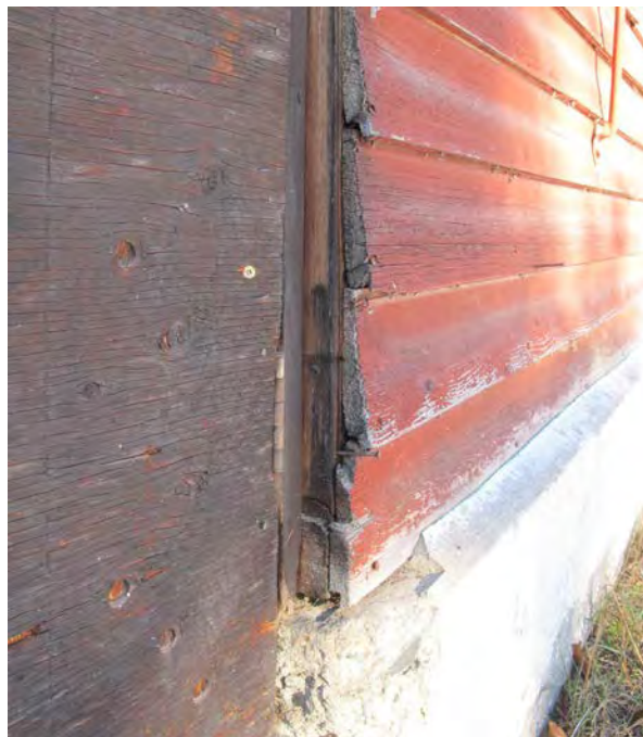
Photos showing typical deteriorated condition of exterior wall cladding above concrete foundation walls. Note profile of original drop siding (top right).
