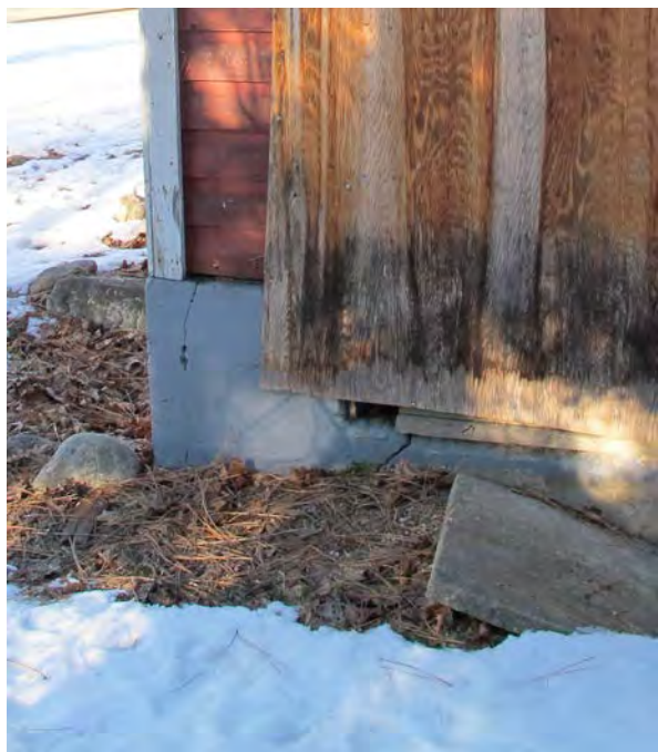
Photos showing typical deteriorated condition of exterior wall cladding above concrete foundation walls. Note profile of original drop siding (top right).
