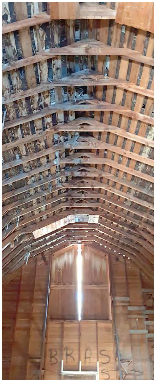
Photo showing interior side of the exterior wood-frame walls, looking north, and underside of the gambrel roof structure of the Surtees Barn.
