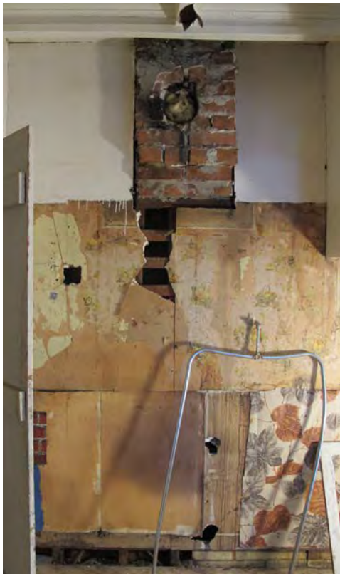
Interior brick masonry chimney flue terminating at midsection of the interior wall, partially showing wood structural support.
