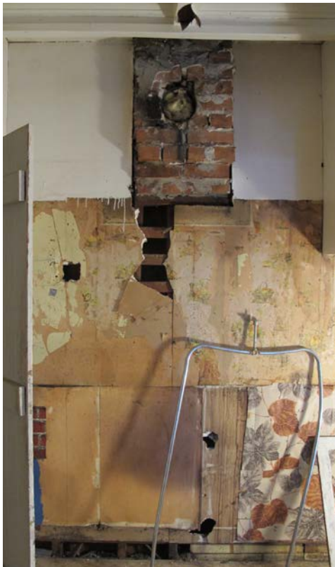
Interior brick masonry chimney flue terminating at midsection of the interior wall, partially showing wood structural support.
