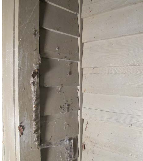
Photo showing existing condition of original exterior wall, with horizontal lapped wood siding and trims at north elevation (top left), and at the interior return walls of the enclosed early addition to the west (top right).
