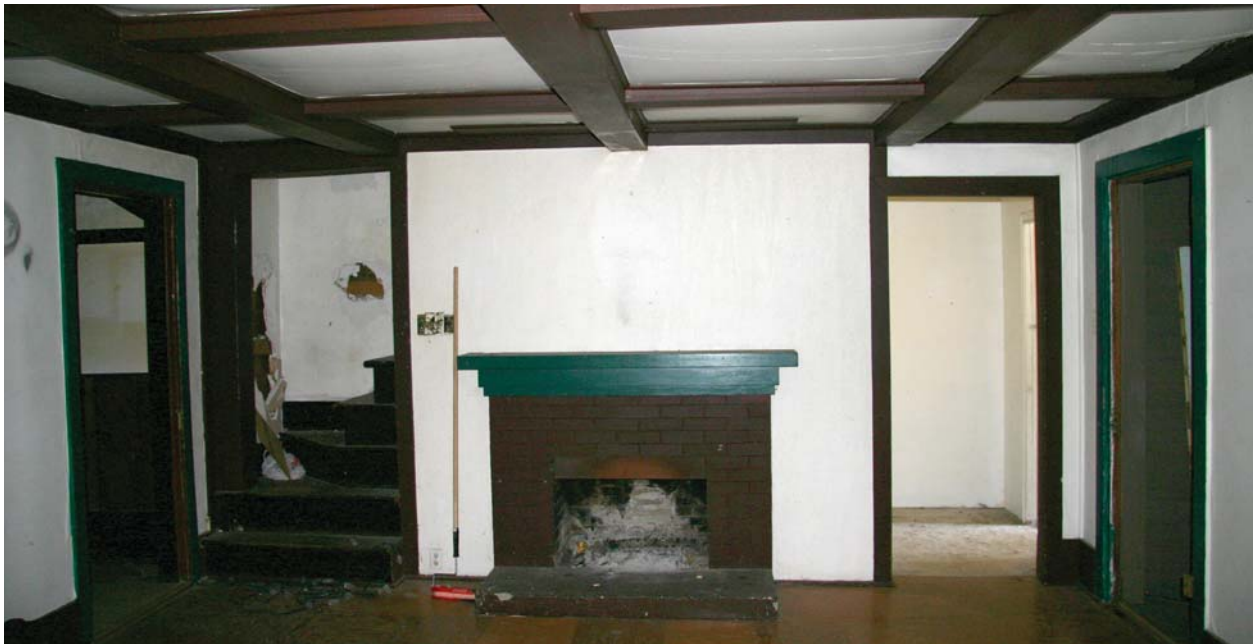
Photos showing surviving interior character-defining elements of Surtees House, including narrow winder staircase; brick masonry fireplace with raised concrete hearth and wood mantel; low ceiling with expressed horizontal beams and coffered-effect.
