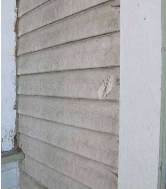
Photo showing existing condition of original exterior wall, with horizontal lapped wood siding and trims at north elevation (top left), and at the interior return walls of the enclosed early addition to the west (top right).
