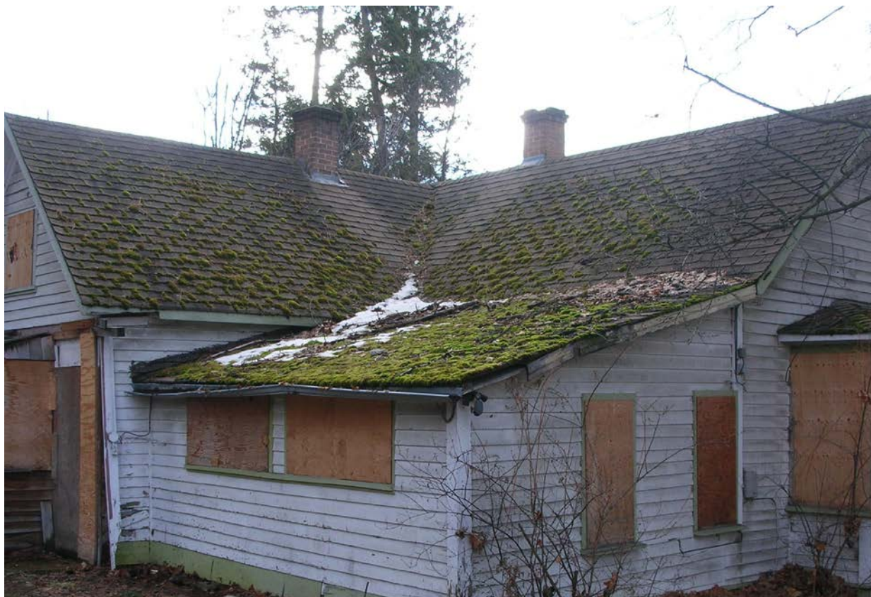
Existing condition of original, primary cross-gabled roof, with shed roof extension of early addition to the northeast portion of the house, as well as two original interior brick masonry chimney stacks along the roof ridges.
