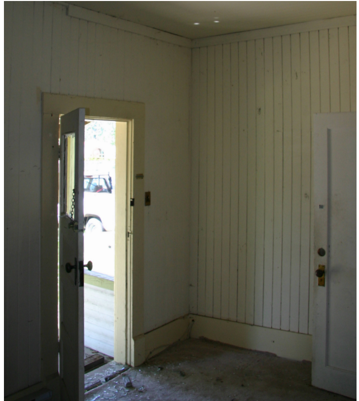
Surviving original v-joint panelling on walls and ceiling of front hall, showing original main entrance door to the left.
