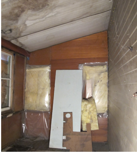
Interior space of the enclosed vestibule (west early addition) showing original exterior horizontal wood lapped siding to the right.
