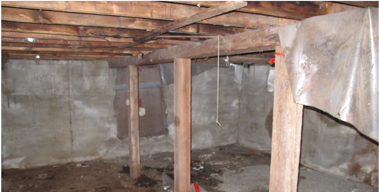
Basement of the west extension to the Surtees Barn.
