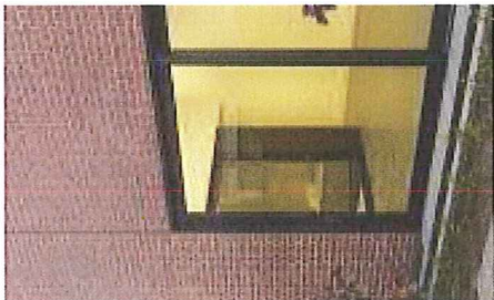
BRICK FINISH WITH DARK WINDOW FRAME
