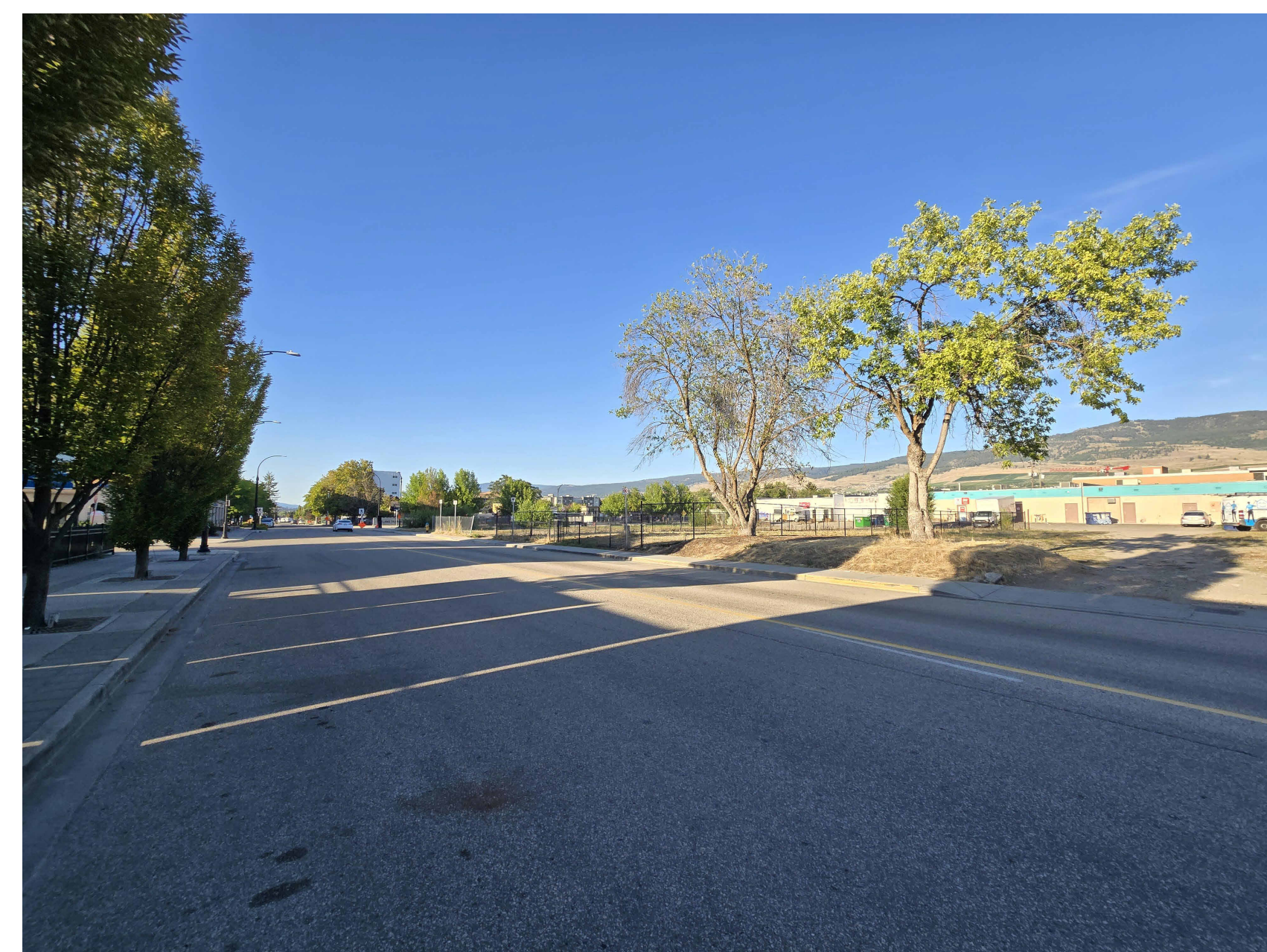
4. VIEW FROM DOUGALL ROAD LOOKING NORTH
