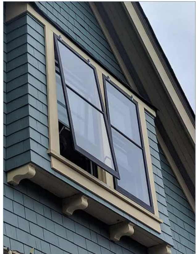
Figure 22: Achieve thermal efficiency by repairing and maintaining existing wooden windows. Installing wood-framed storm windows can further improve thermal efficiency and provide sound abatement.
