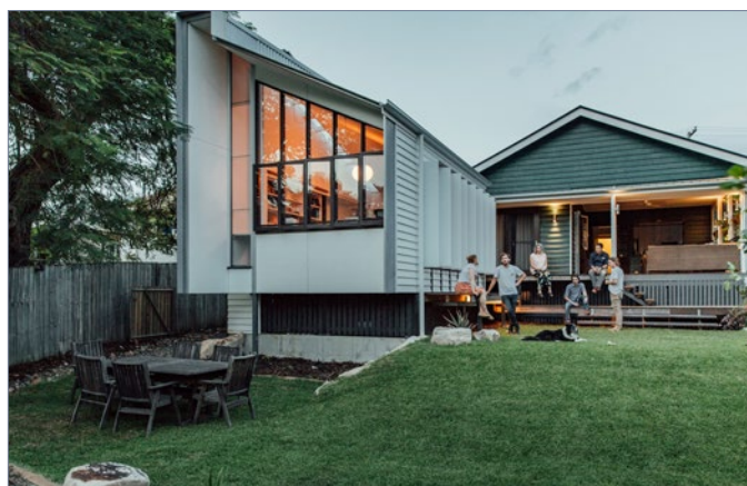
Figure 12: Use durable, fire-resistant, or non-combustible materials for new properties within the HCAs, including smooth finished fiber cement siding and shingles, fiber cement panels, stucco cladding, and metal cladding.
