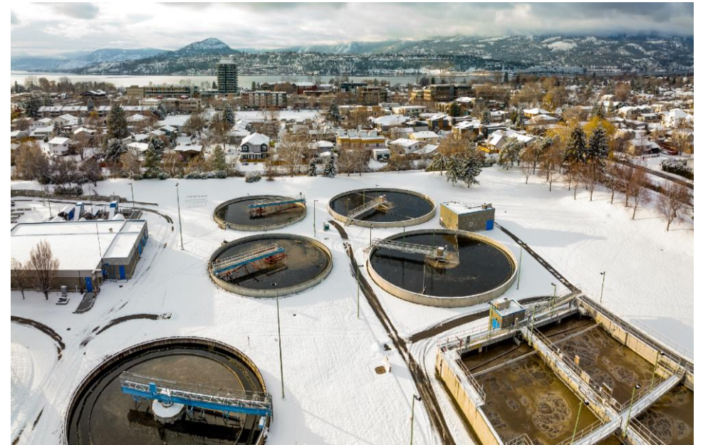
Secondary Clarifiers Raymer Wastewater Treatment Plant
