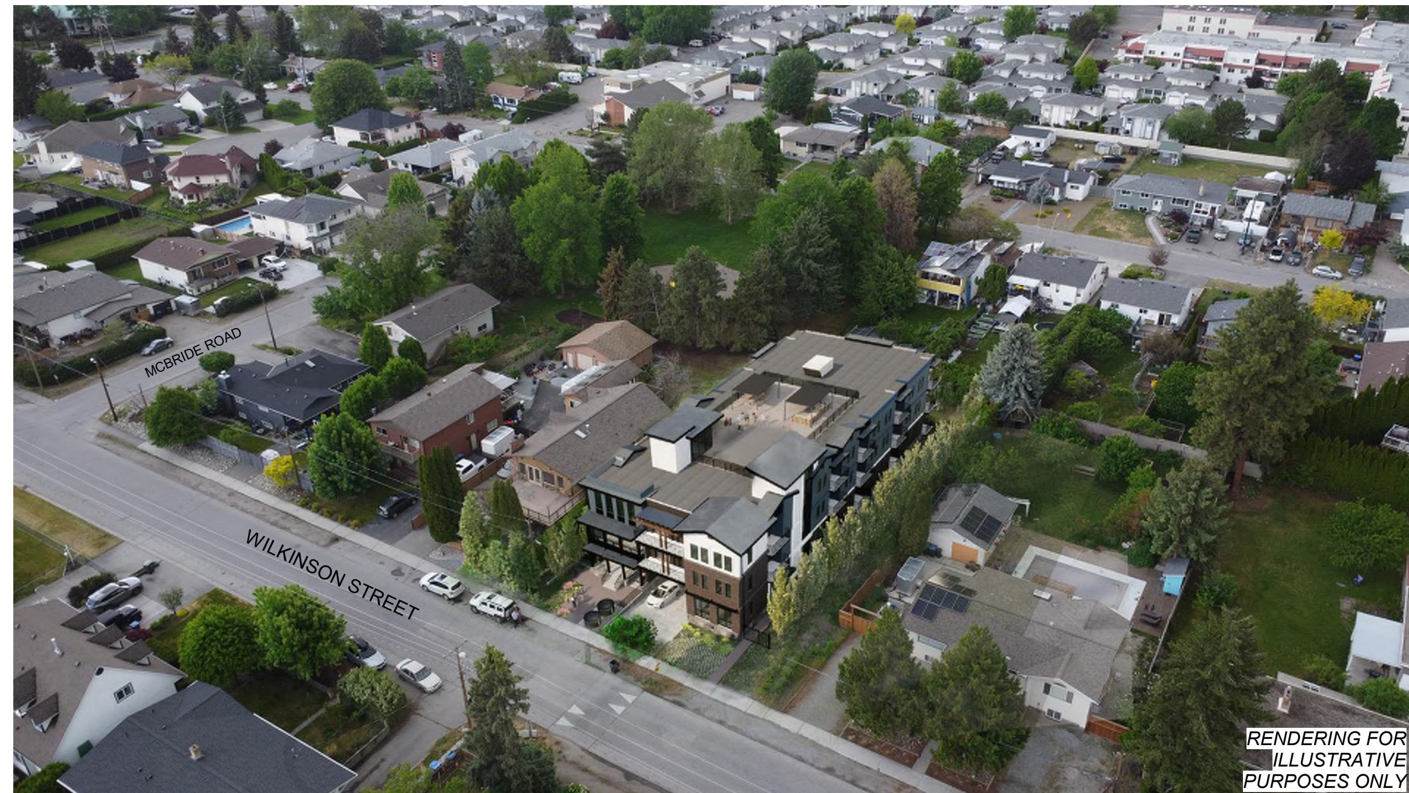
AERIAL CONTEXT VIEW FEATURING PARK
