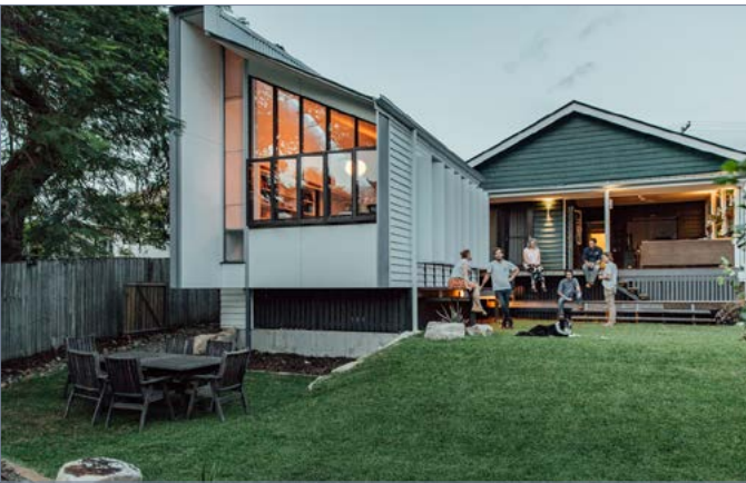
Figure 12: Use durable, fire-resistant, or non-combustible materials for new buildings within the HCAs, including smooth finished fiber cement siding and shingles, fiber cement panels, stucco cladding, and metal cladding.
