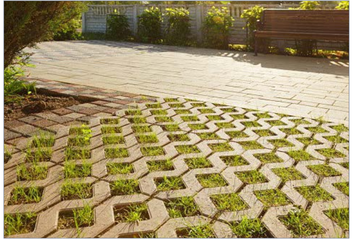
Figure 26: Improve runoff quality onsite using best practices, such as draining to vegetation, using permeable paving and/or collect and drain runoff.
