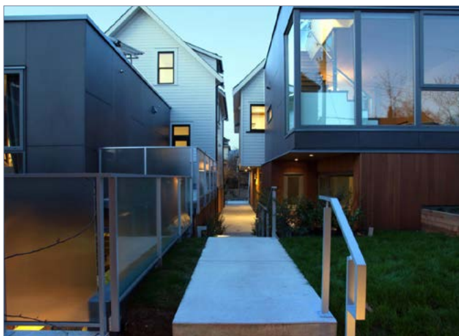
Figure 10: Use links, breezeways, insets, or offsets for side and rear additions to connect to the historic building, distinguishing their massing from the original house.
