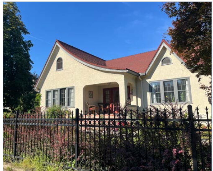
Figure 15: Retain, repair, and restore original doors, transoms, sidelights, and hardware whenever feasible.
