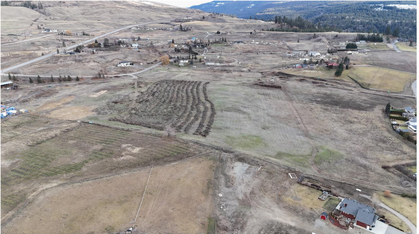
Photo #1: December 2023 aerial image of soil and fill placed and ready to be spread from North (left) to South (right).
