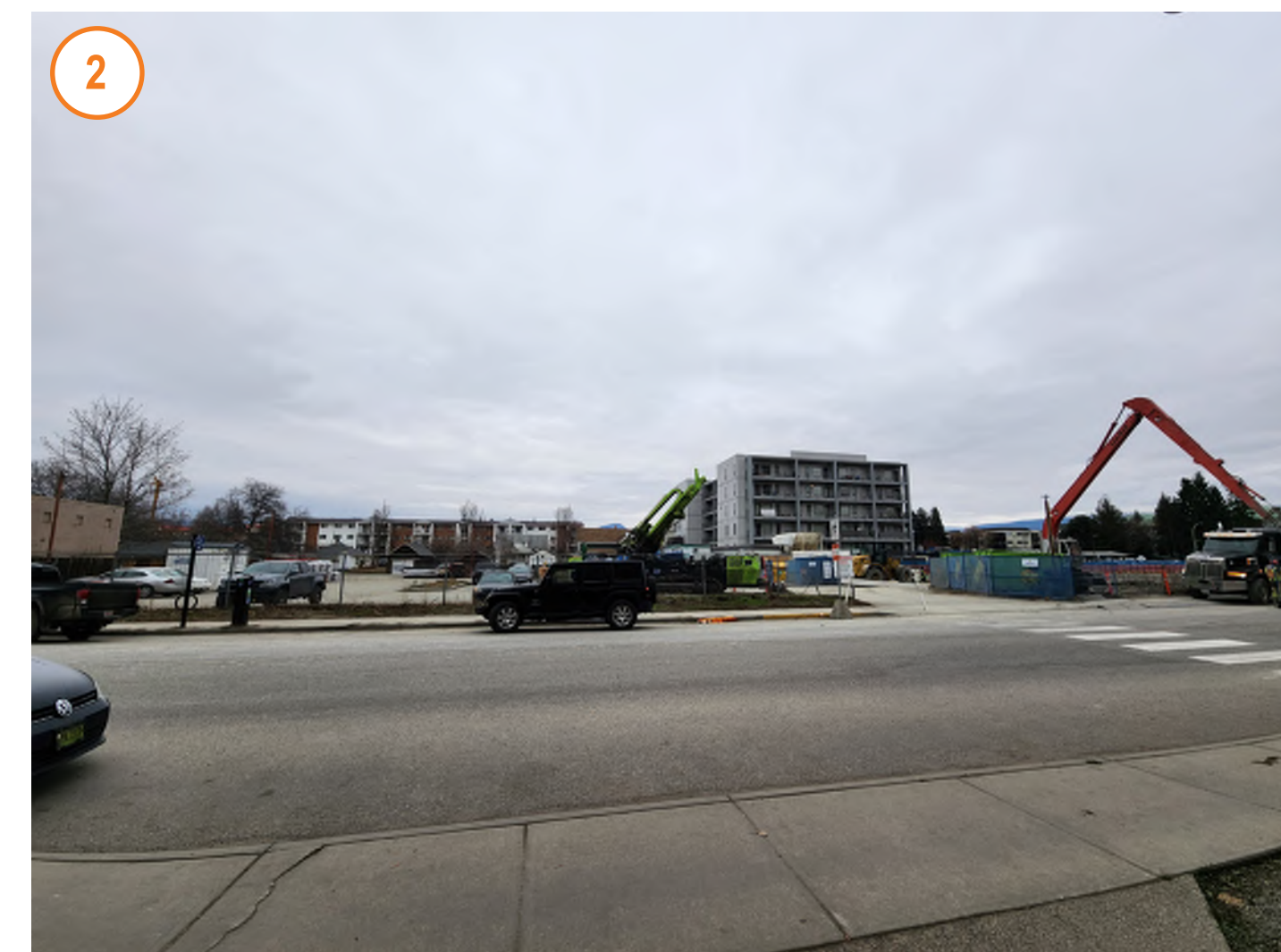
View facing East along St.Paul St
