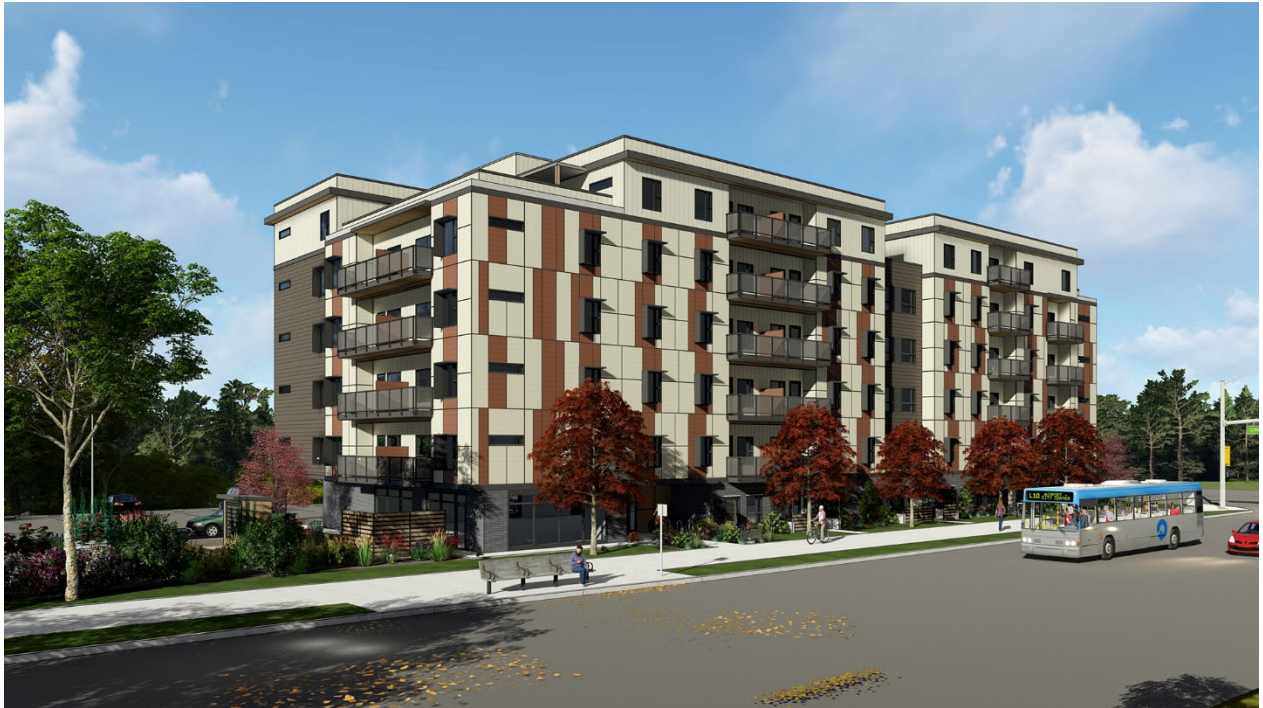
Figure 1: View from Glenmore Road
