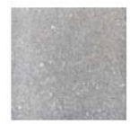
H11 SAND BLASTED CONCRETE
