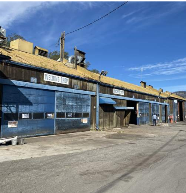
Figure 70. Exterior view of the Machine Shop
