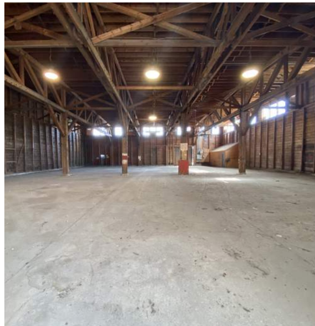
Figure 67. Inside No. 5 Shed
