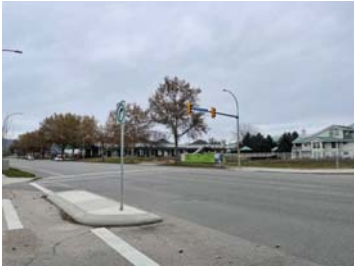
C EXIST. VIEW FROM GORDON & CAMERON, LOOKING NORTH EAST
