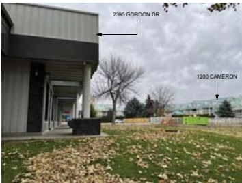
E EXIST. VIEW FROM GORDON, LOOKING EAST
