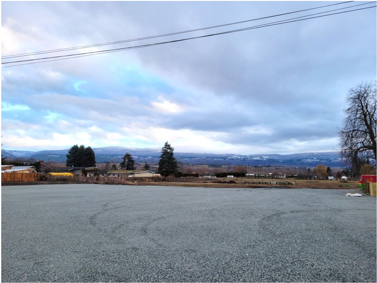
Photograph showing the original soil and rock storage area cleaned up.
