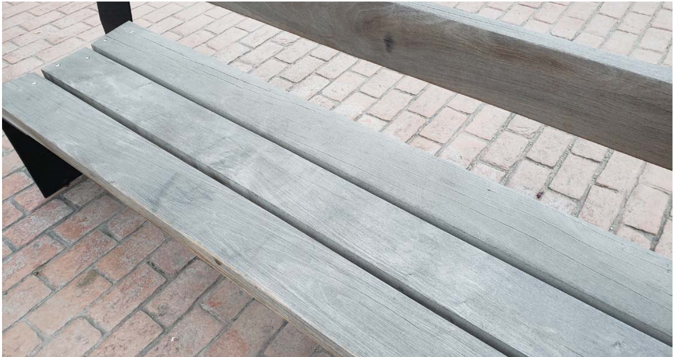
Figure 22: Timber checking on rear bench slat
