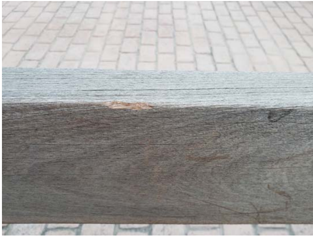
Figure 20: Chip damage on timber backrest top slat of bench
