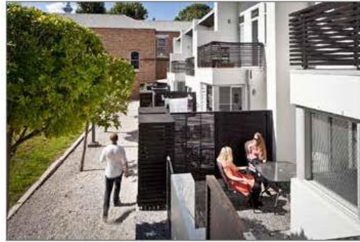
Figure 22: All units should have easy access to useable private or semi-private outdoor amenity space (3.1.4 a).
