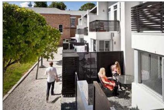
Figure 21. All units should have easy access to useable private or semi-private outdoor amenity space (3.1.4 a).
