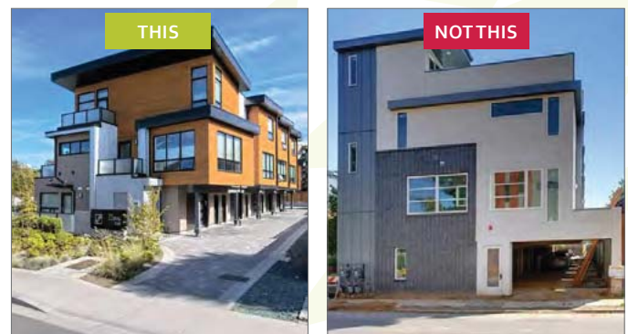
Figure 18: In 'shotgun' townhouse projects, ensure that the end unit facing the street is a true street-oriented unit (3.1.1 d).
