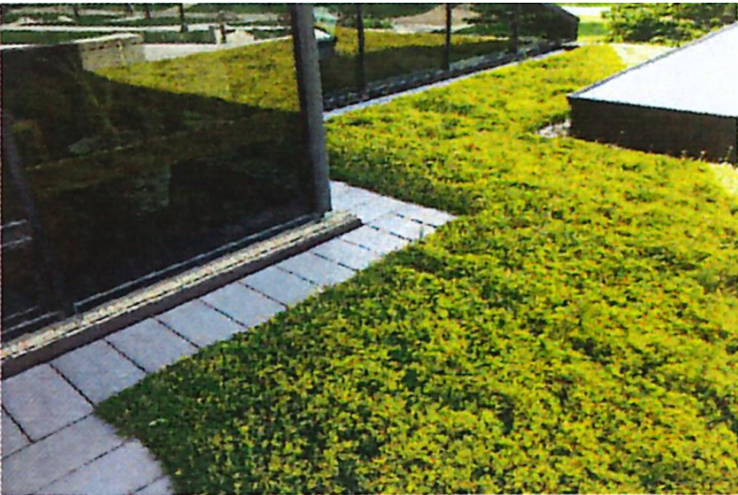
EXTENSIVE GREEN ROOF
