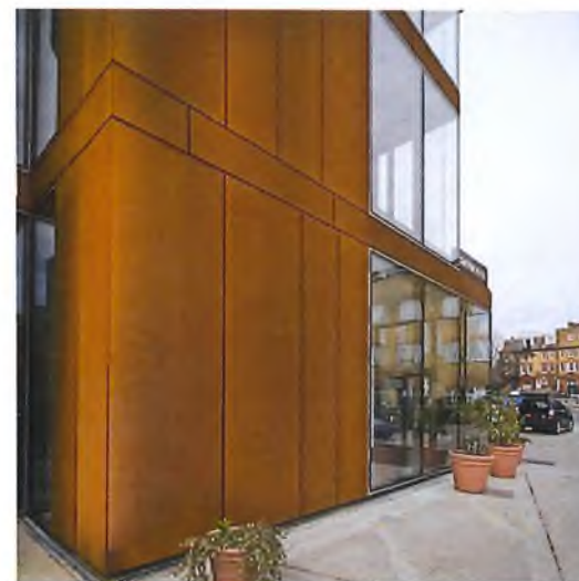
WEATHERING STEEL CORTEN
