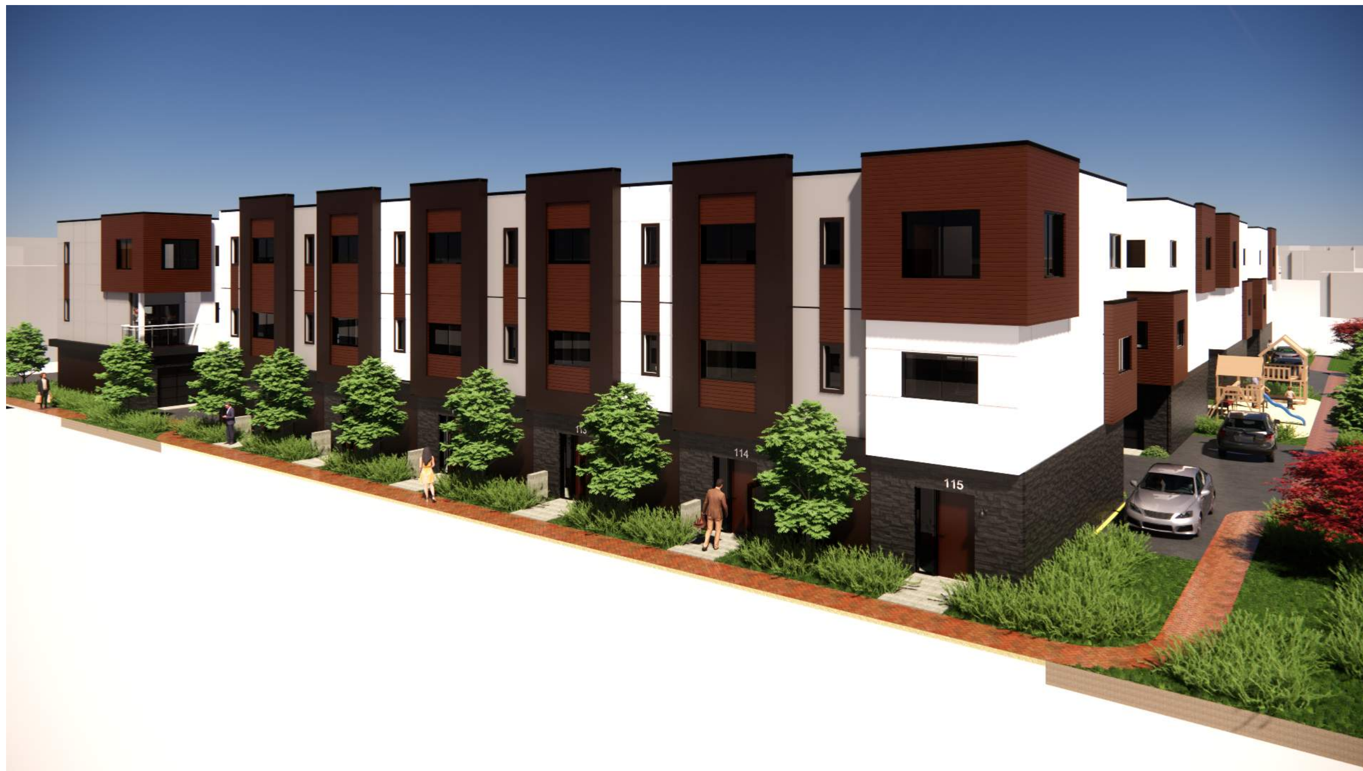
#3 - BUILDING #6 (NW CORNER)
