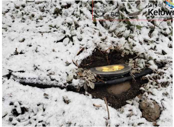
Figure 9: Exposed irrigation line visible in raised planter near uplight.
