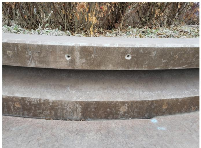
Figure 12: Holes in wall of raised planter
