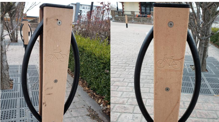
Figure 23: Scuffing and wear on bike rack posts
