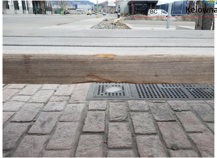
Figure 21: Chip damage on front of timber bench slat
