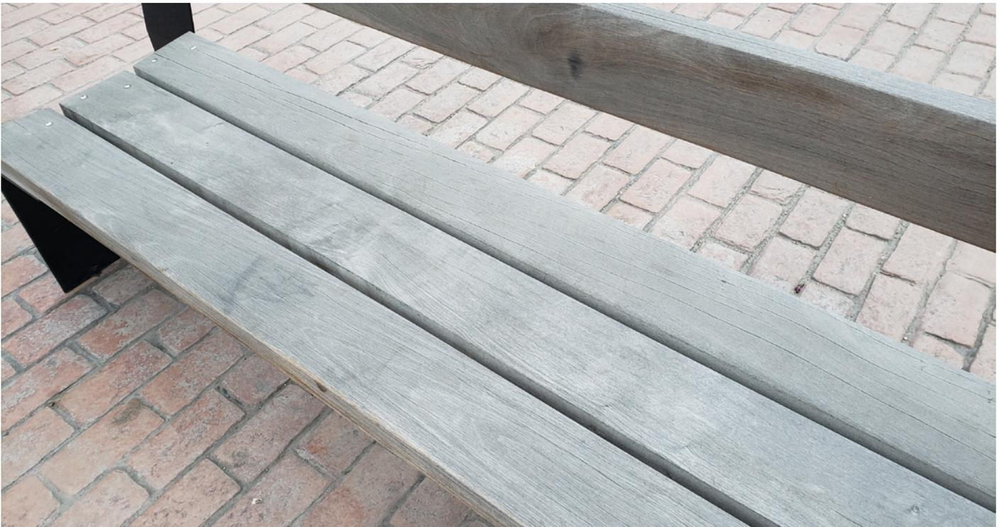
Figure 22: Timber checking on rear bench slat
