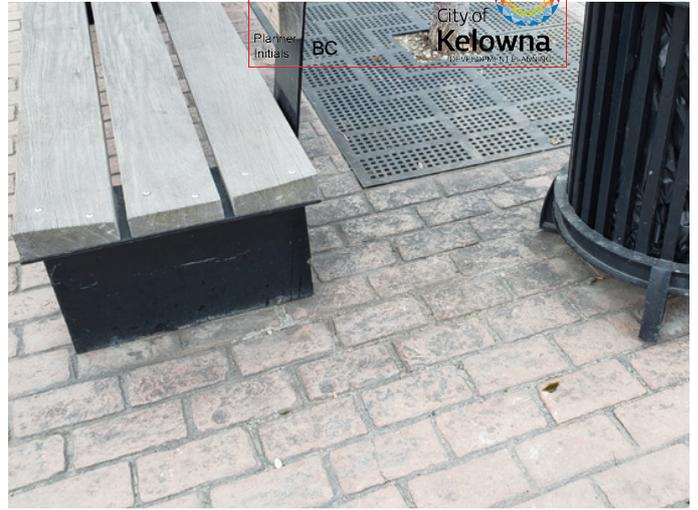
Figure 26: Darkening on stamped concrete paving
