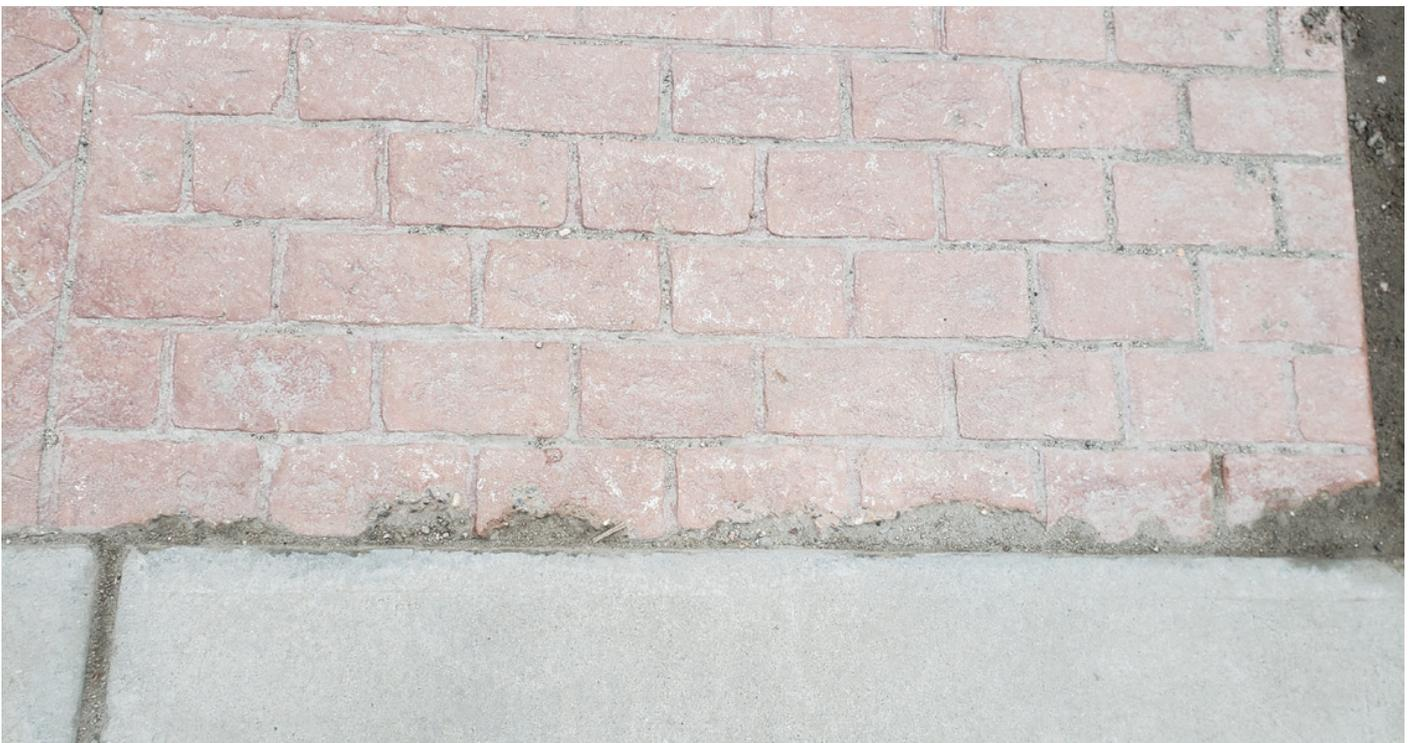
Figure 15: Cracking of stamped concrete paving along edge of municipal sidewalk at Southeast corner of garden, off Clement Avenue
