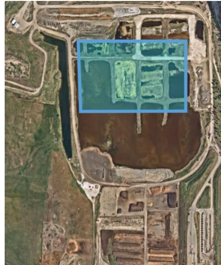
BURNT WASTE PILES
