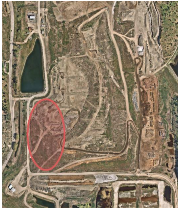
LANDFILL GAS DAMAGE AREA
