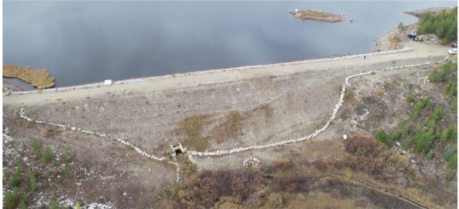
Figure 2-22: Turtle Lake South Cut-off Dam – Oblique photograph of dam (October 2021)
