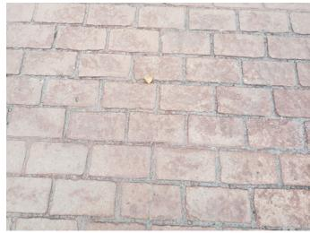
Figure 16: Small crack in surface of stamped concrete paving
