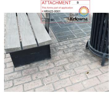
Figure 26: Darkening on stamped concrete paving
