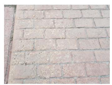
Figure 28: Salt damage along East side of plaza
