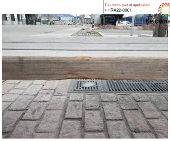
Figure 21: Chip damage on front of timber bench slat
