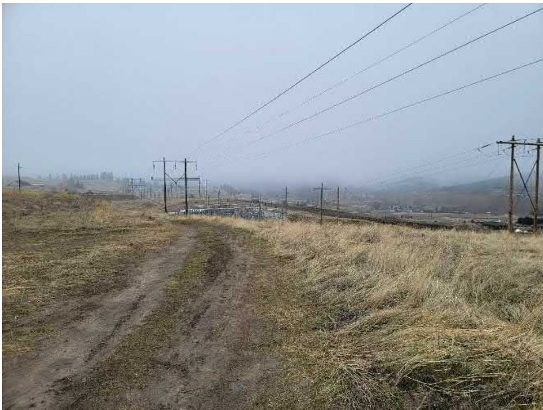
Photo 1.24: Site access and overhead electrical transmission lines west of the fill placement area
