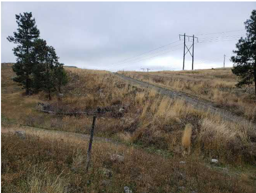
Photo 1.2: Northwest fill placement limits and adjoining access road
