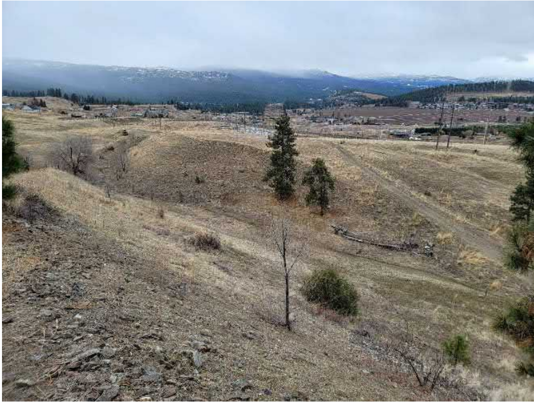
Photo 1.7: View of the fill placement area looking southwest from the steep side slope
