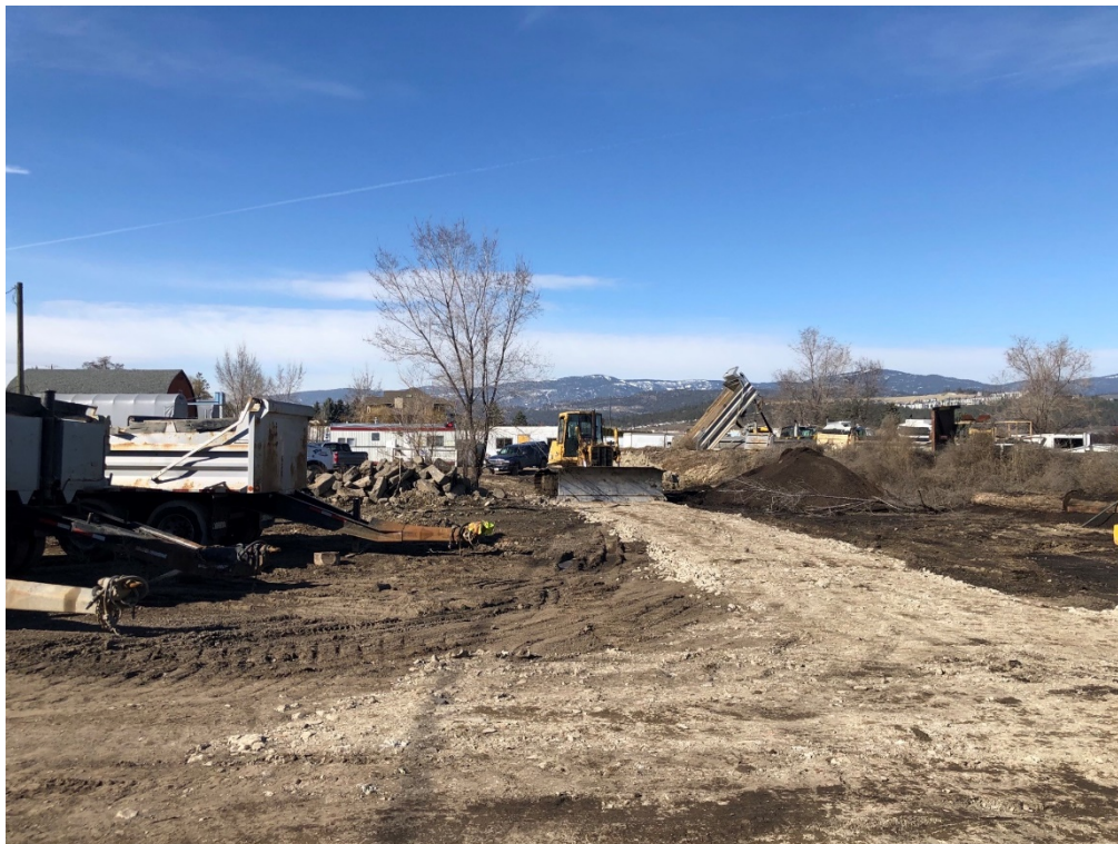
Photo 5. View of machinery and site office in the background
