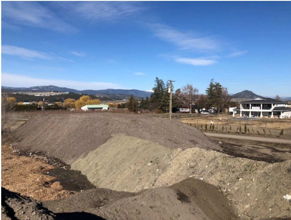
Photo 6. Berm constructed to reduce noise pollution
