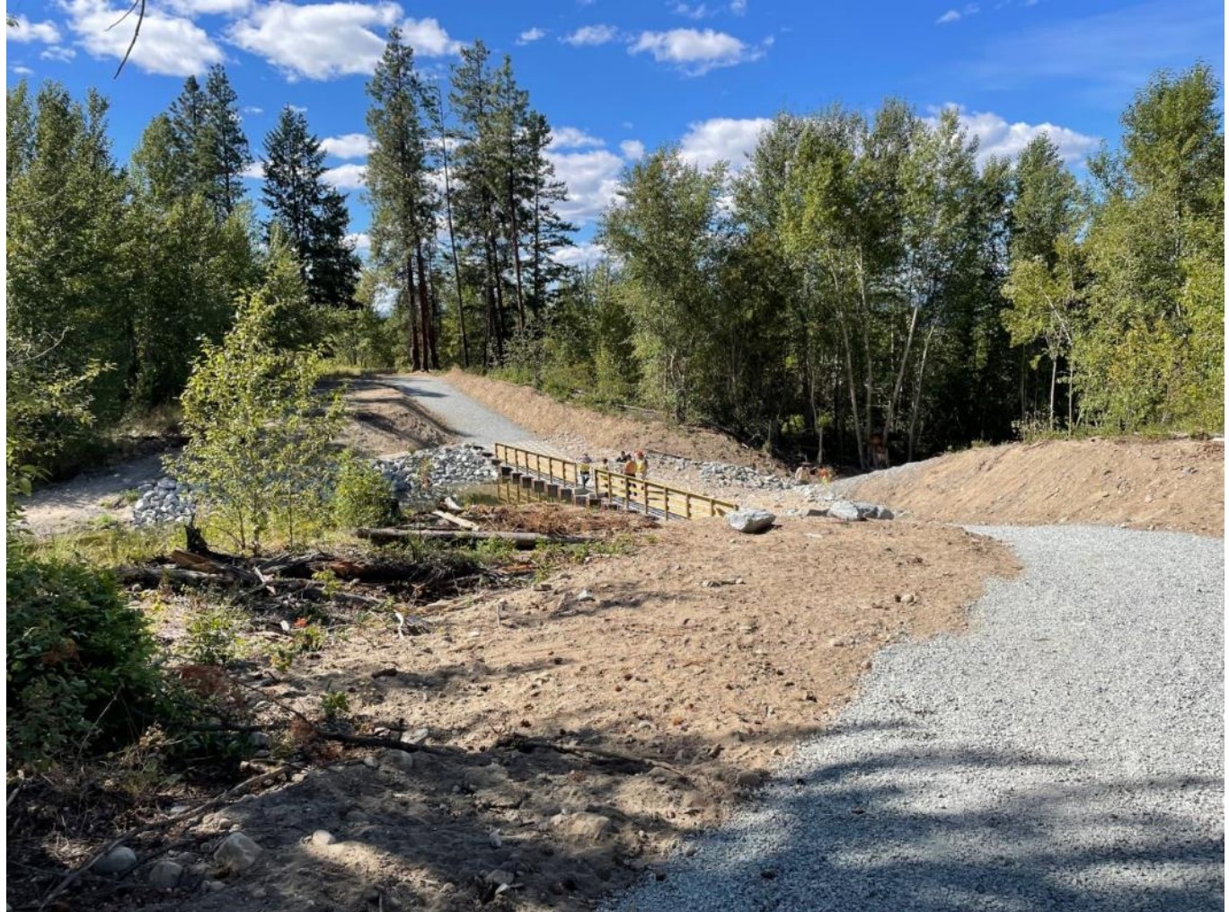
The new Frazer Lake Dam
