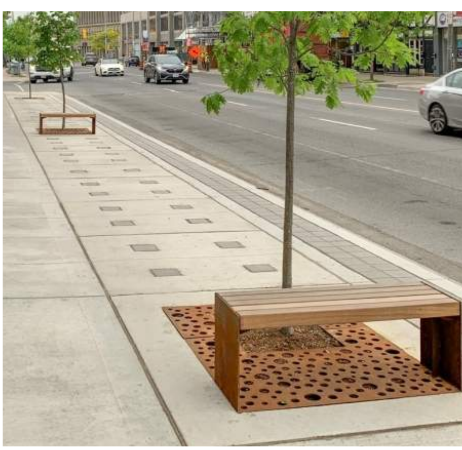
TREE GRATE WITH BENCH PRECEDENT IMAGE FOR TREE GRATE BENCH LAYOUT (SEE PROJECT BENCH NOTED BELOW FOR PROPOSED PRODUCT)
