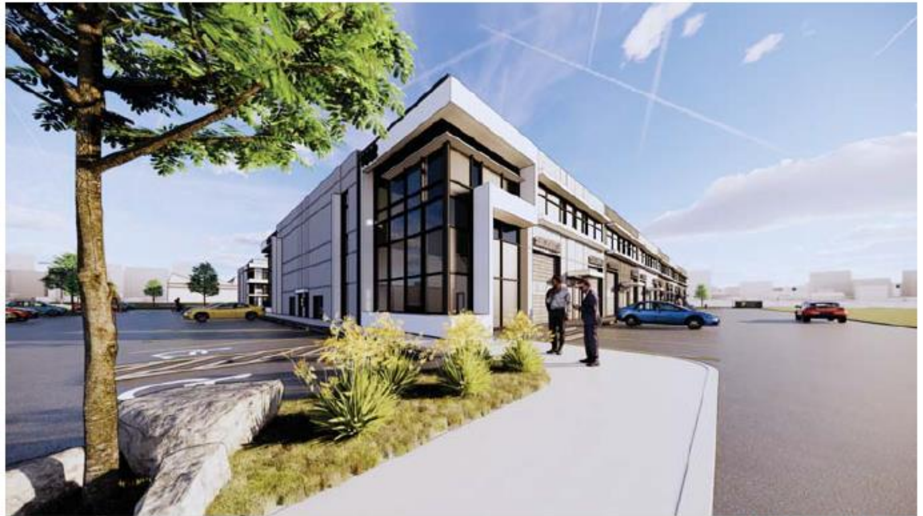
VIEW FROM NORTH ENTRANCE
