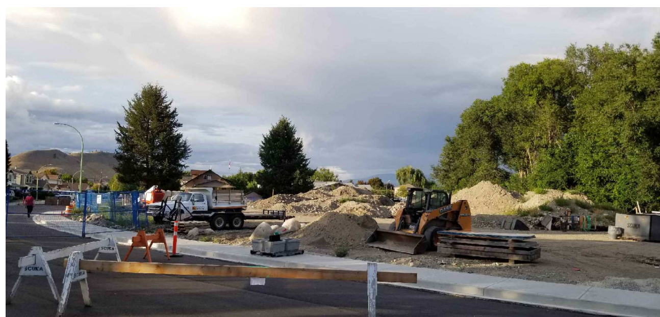
4 PHOTO 2 (2019) VIEW LOOKING NORTH TO SITE
