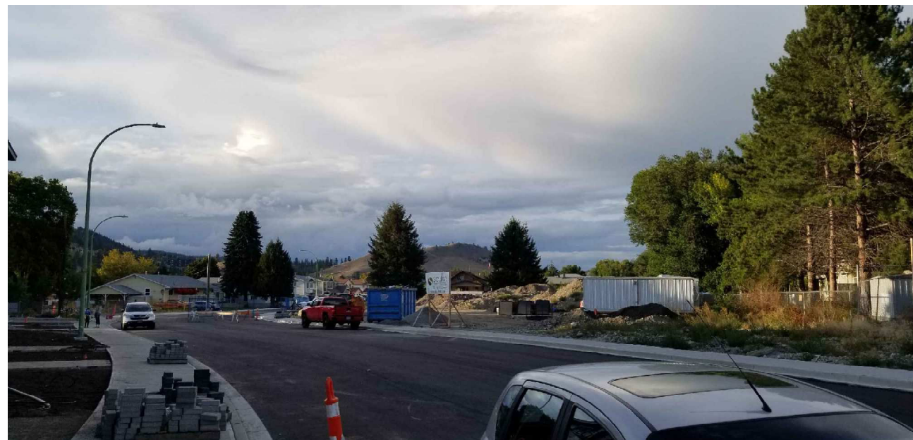
4 PHOTO 3 (2019) VIEW LOOKING NORTH TO SITE
