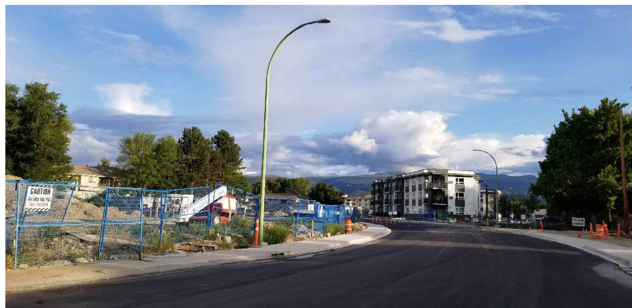
3 PHOTO 1 (2019) VIEW LOOKING SOUTH TO SITE & NISSEN CROSSING
