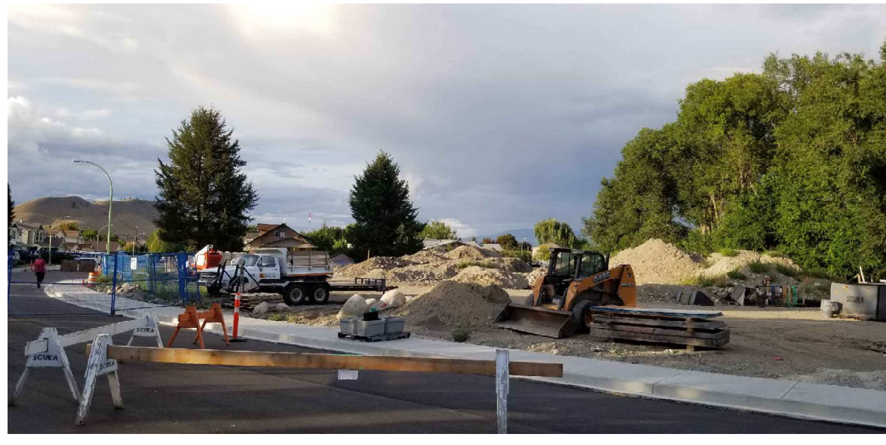
4 PHOTO 2 (2019) VIEW LOOKING NORTH TO SITE
