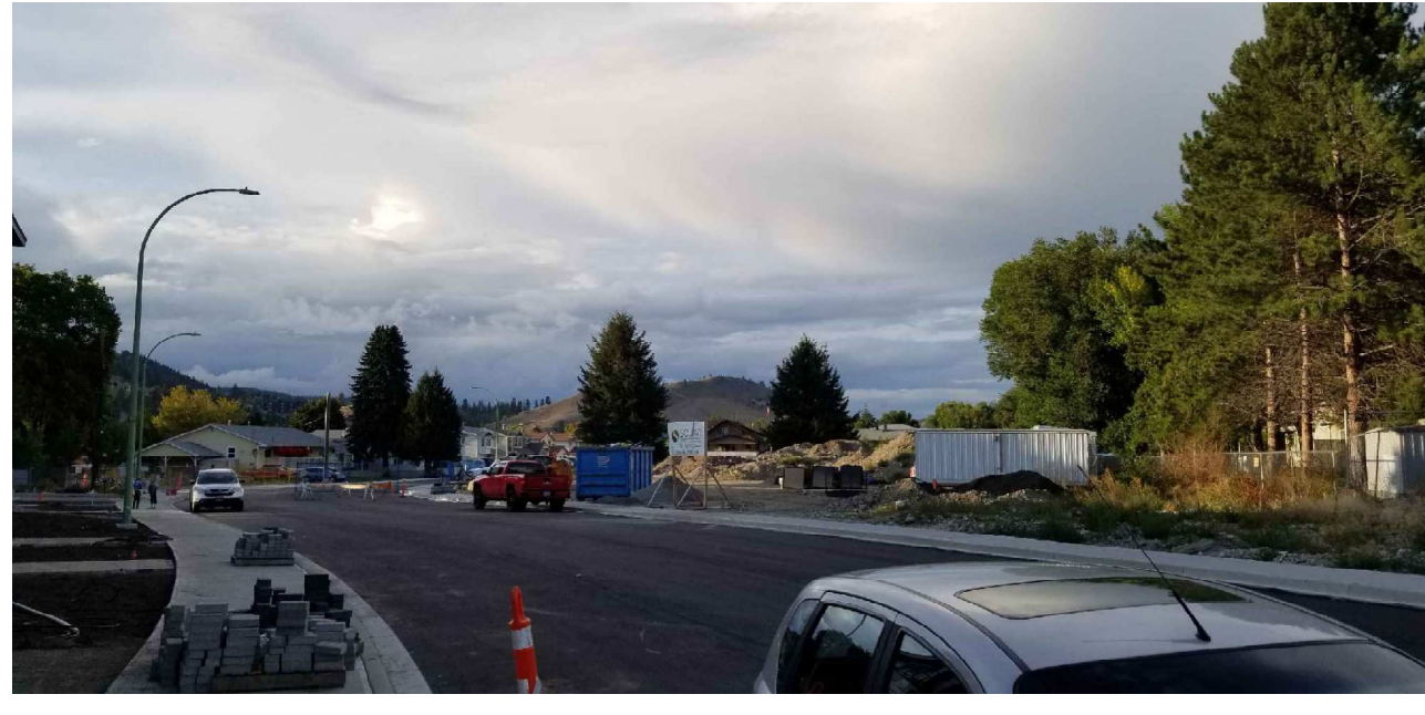
4 PHOTO 3 (2019) VIEW LOOKING NORTH TO SITE
