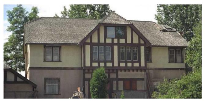
At some point, the house sustained fire damage that was confined to the north-east corner of the home. Ongoing repairs to that damage as well as roof maintenance continue presently. The applicant received a Heritage Grant in Central Okanagan Heritage Society to complete the roof restoration with rare yellow cedar shingles that are only in production intermittently and are seasonally dependent. The grant has been extended and is currently valid for the ongoing repairs.
