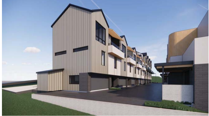
UPBANK UNITS - SOUTHWEST SIDE
