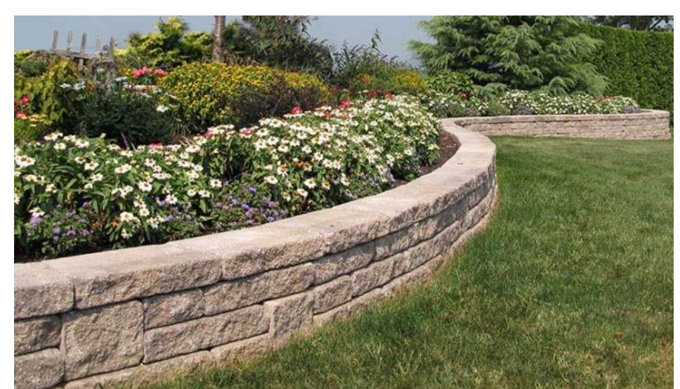
PRECAST BLOCK PLANTER Allan Block Splittfaced Planters On Slab (or Approved Equivalent)
