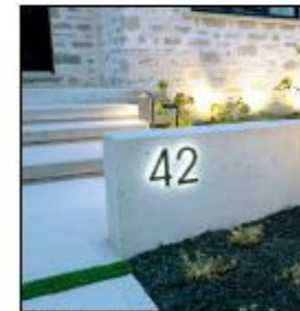
HOUSE NUMBER & CONCRETE WALL
