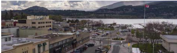
07. View looking toward site looking down from Queensway.
