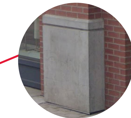
Masonry Details (Precast Concrete)
