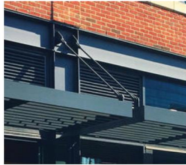
RETAIL STOREFRONT CANOPY DETAILING: 3.: METAL C-CHANNEL FRAMING / METAL BREAK-SHAPE – COLOUR: BLACK 6.: METAL TRELLIS CANOPY (C/W TIE- BACK RODS AS SHOWN) – COLOUR: BLACK 7.: MECHANICAL LOUVER PANEL – COLOUR: BLACK
