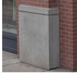
5.: PRECAST CONCRETE WALL BASE LOCATED AT BRICK PILASTERS, C/W REVEAL LINES.
