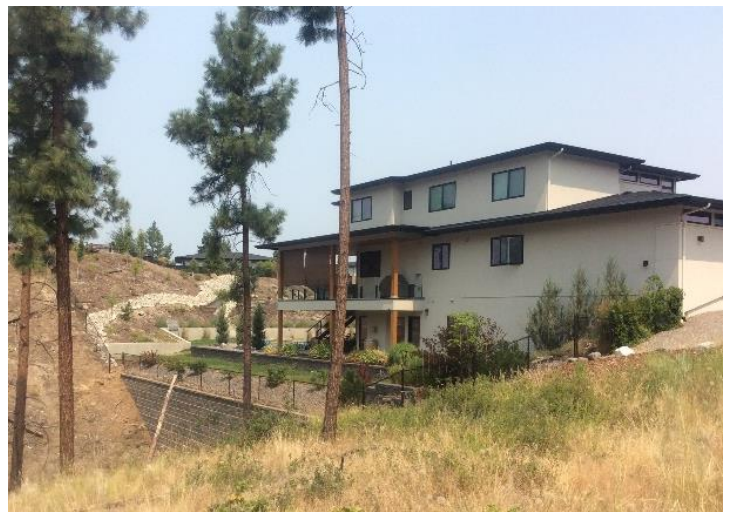
Figure 4. Home located in interface neighborhood in Kelowna with a FireSmart gravel strip at the property line
