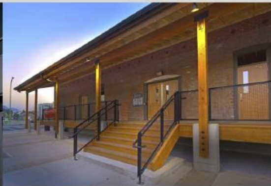
stained wood post and concrete base with good lighting
